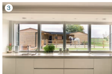
1 A traditional configuration sees side-opening casements vertically aligned with top-hung sections, like this example by Westbury Windows & Joinery. The top portion is opened for gentle ventilation 2 Fakro's wood-vener FPP-V model is ideal for loft conversions and other pitched-roof sites 3 Top-guided windows, like these triple-glazed Velfac examples used in a Cambridgeshire house, give better ventilation than a straightforward top-hung model, because they open up an extra gap at the top
