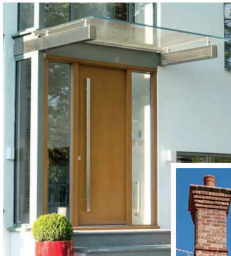
Left: Building Regs say that glazed areas within 800mm of the floor, such as the sidelights on this front door by Kloeber, should be fitted with safety glass
