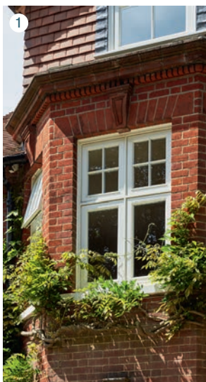
1 A traditional configuration sees side-opening casements vertically aligned with top-hung sections, like this example by Westbury Windows & Joinery. The top portion is opened for gentle ventilation 2 Fakro's wood-vener FPP-V model is ideal for loft conversions and other pitched-roof sites 3 Top-guided windows, like these triple-glazed Velfac examples used in a Cambridgeshire house, give better ventilation than a straightforward top-hung model, because they open up an extra gap at the top
