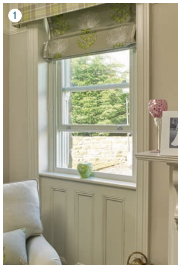
1 This triple-glazed timber unit by Green Building Store is spring-balanced, and costs from £1,150 2 Traditional timber sashes in a dormer, by Westbury Windows & Joinery; available either sprung-balanced or with a weight and pulley mechanism 3 Rehau's PVCu sliding sash does a good job of replicating the detail of its timber predecessors and it's A-rated for energy efficiency
